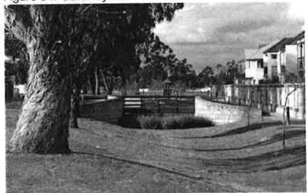
Figure 56. Footpath crossing swale
